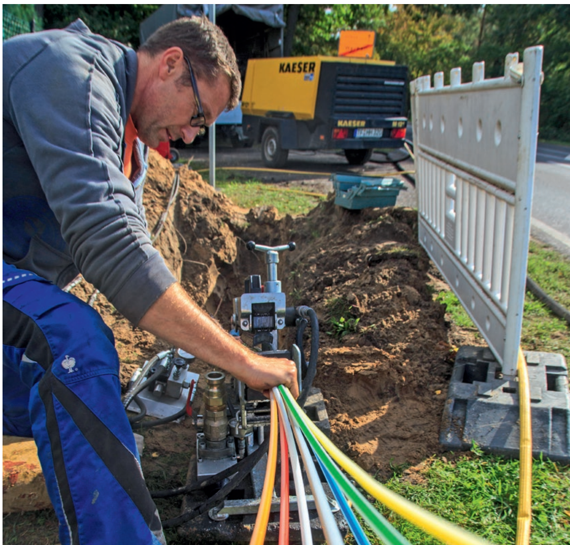
Ostprignitz-Ruppin: Empty conduits for fibre optic cables are inserted into a thick underground cable and subsequently fitted with fibre optic bundles. Brandenburg will continue to push ahead with the roll-out of fibre optics in the coming years.
